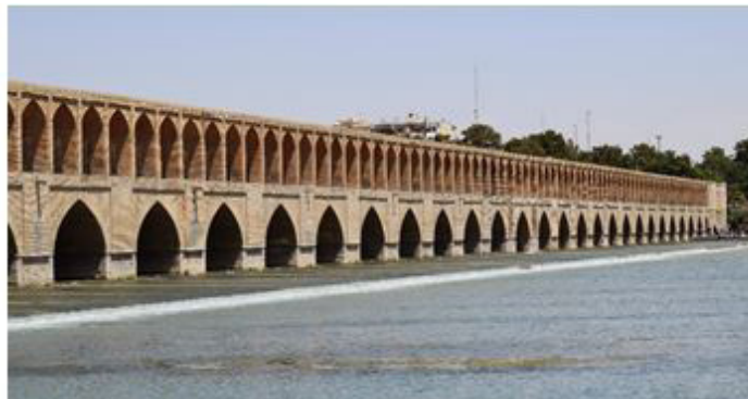
Fig.1: Allahverdi khan bridge
