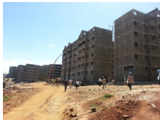
Fig. 6: House type at Redevelopment site for Kibera settlement
