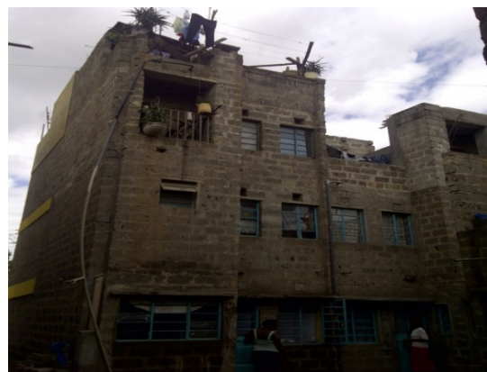
Fig. 8: House type under construction at Kambi Moto Settlement
