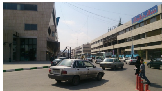
Fig. 5: Square Exterior Chambered, Toos: Building
