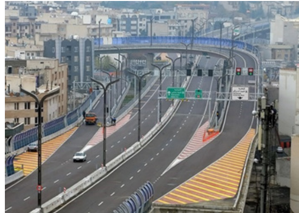
Figure 4: Discontinuity of Sadr elevated highway noise barriers (Ghorbani, 2013)
